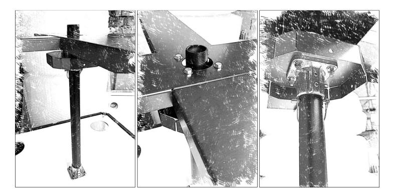
Place the other Frame Cross Beam over the top of the other beam so that they cross each other. Line up the 4 holes as best you can and insert the 5/16<sup>th</sup> bolts with washer through the holes. Be patient and do one bolt at a time. Once you get all 4 bolts through, go ahead and add the other washers and nuts. Tighten it down firm enough so the bolts don't spin but not so tight that the metal bends.
